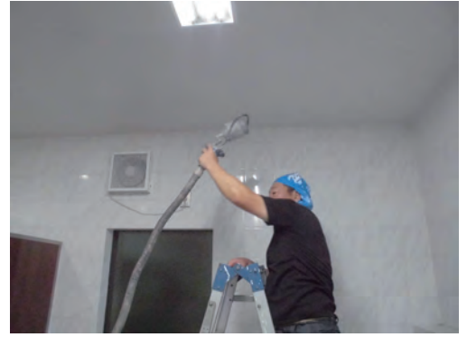
Faith guard-inAttack3を壁面・天井に塗布
