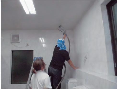
Faith guard-inAttack3を壁面・天井に塗布
